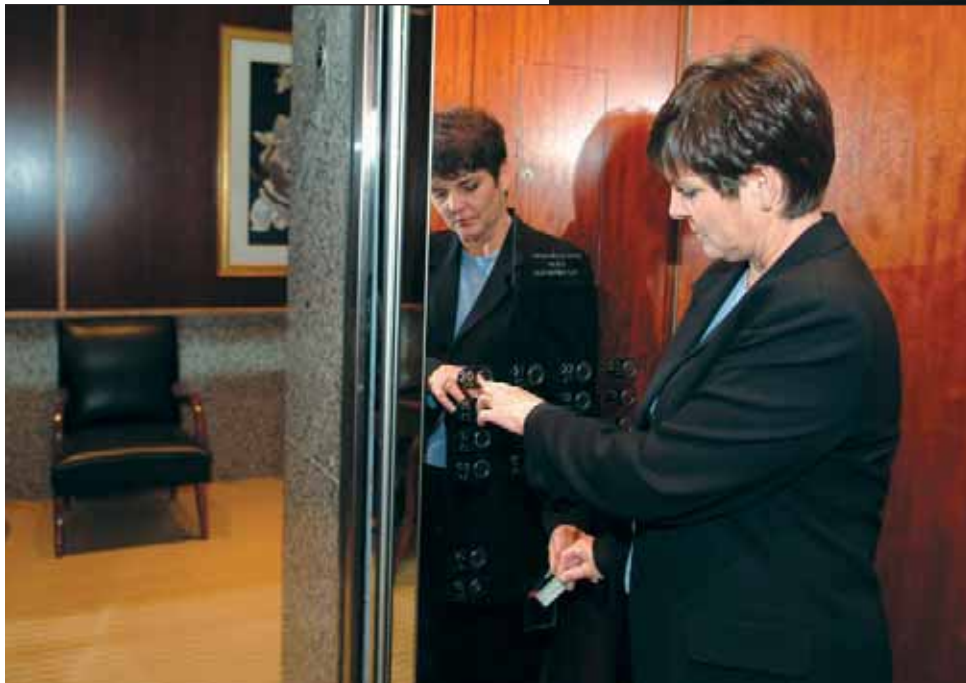
Left, open architecture was the aim of electronic access control systems at Stiles Property Management of South Florida, says Judy Carter, senior property manager. Right, an automated elevator system at the Bank of America Plaza at Las Olas Centre where a small screen on the elevator door confirms the person's floor stop after using a proximity system or keypad.
